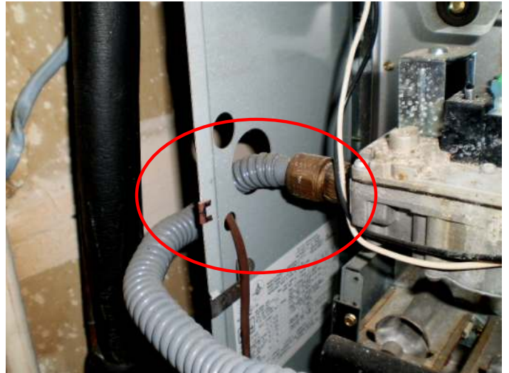
Sample picture of the correct installation of the heating unit flex connector.
