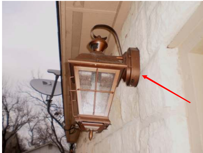
Exterior light fixtures should be sealed to the structure.
